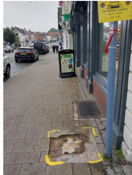
Photo 3 – Photograph the defect and the view down the road/pavement
